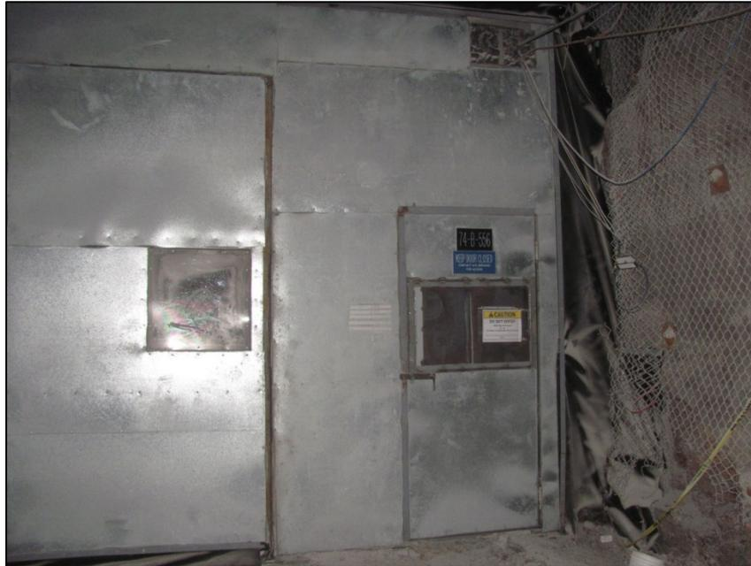
Figure C-2 - Bulkhead with Vehicle and Man Doors
