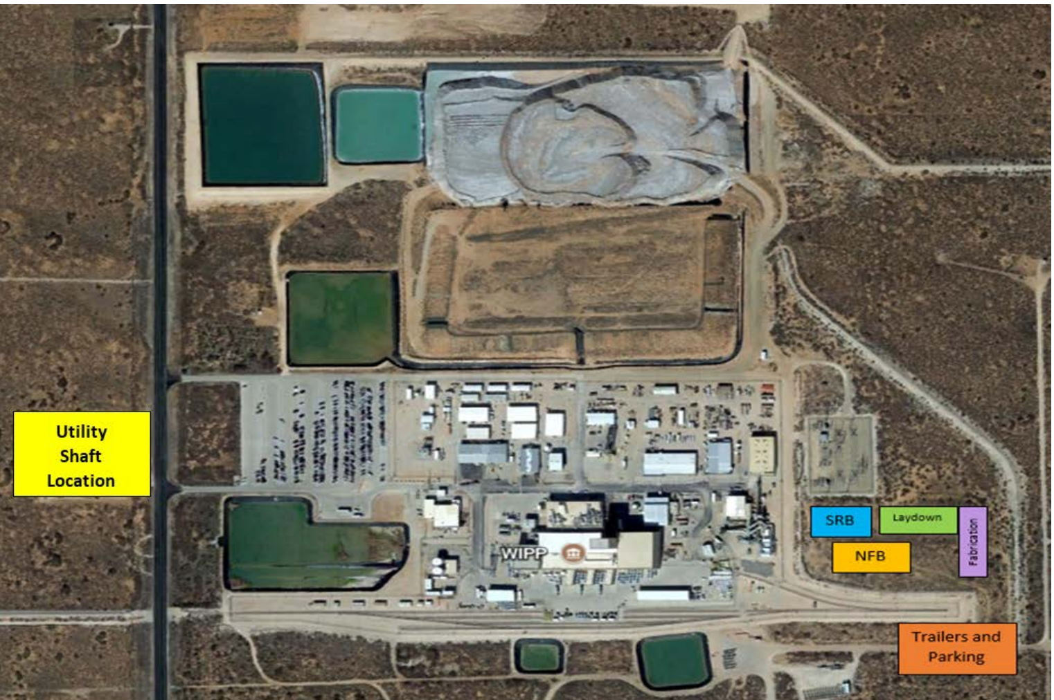
Figure 2.4-3. WIPP Surface Structures with Utility Shaft
