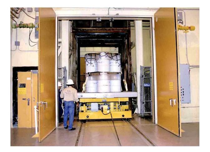
Figure B4-7 Waste Shaft Conveyance - Loading Facility Pallet with CH Waste, Waste Handling Building
