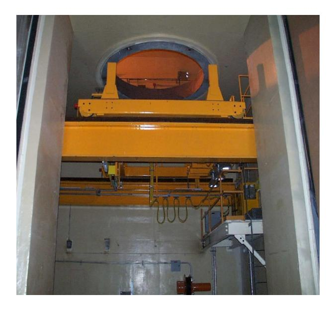
Figure B4-9 Cask Unloading Room and Bridge Crane
