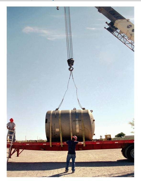
Figure 2.3-13 – Horizontal Lift and Securement of a TRUPACT-II Using Weld-On Lugs
