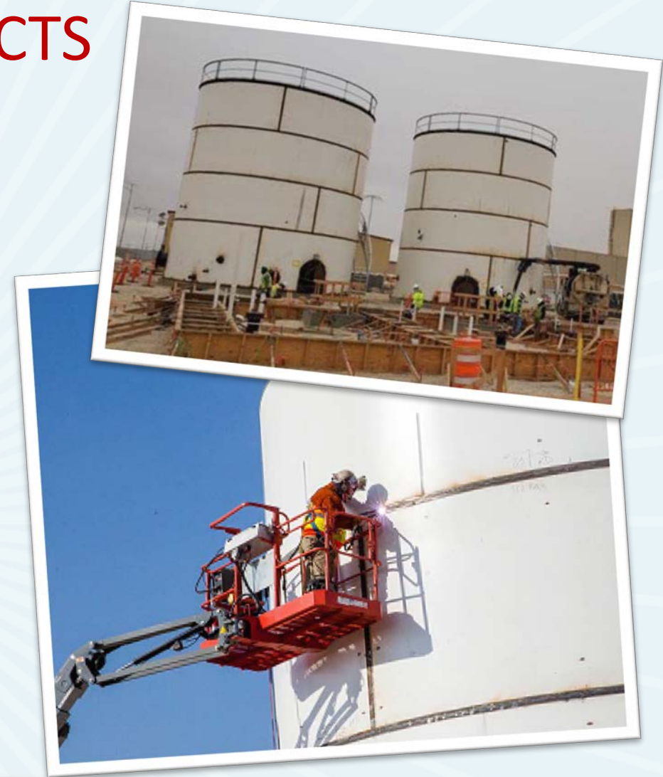
Construction of the new Fire Water Tanks for the Fire Water Loop System
