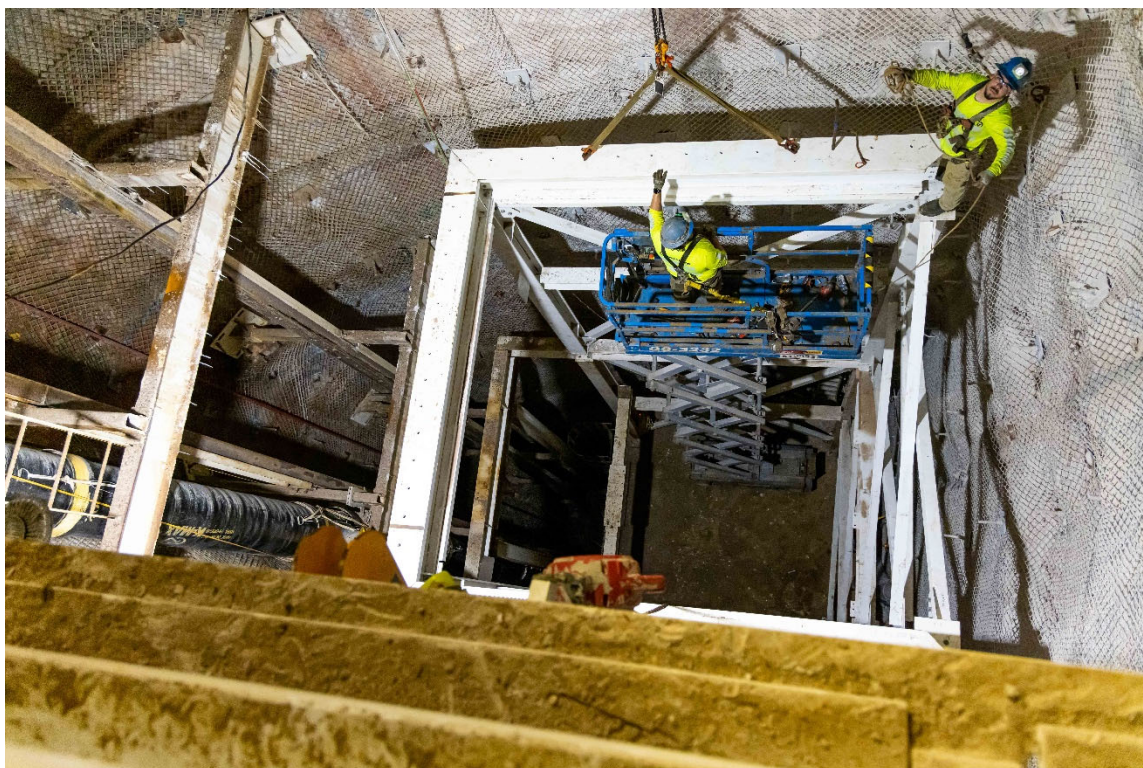
Figure 2.0 – The Salt Hoist Pocket Project
