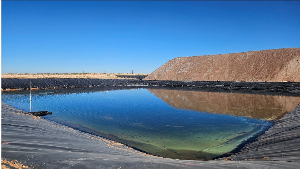
Figure 2.1 – SSP 2 Liner Replacement
