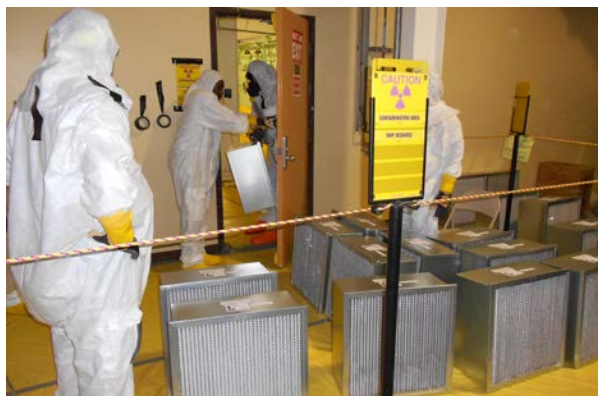
Radiological workers ready used filters for off-site disposal.
