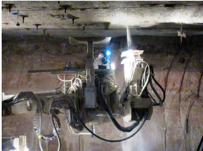
**An Underground Operations employee, wearing anti-contamination clothing and a respirator, installs bolts in Panel 7 of the WIPP underground.**
