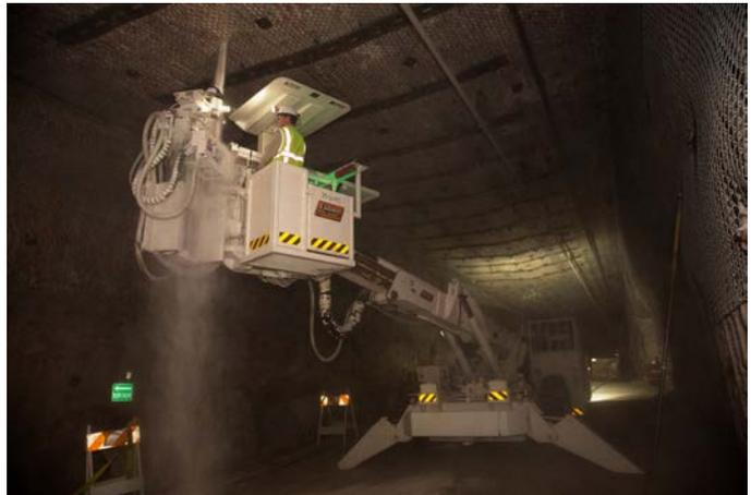
An underground operations worker uses the one of the new hybrid bolting machines to drill a hole in preparation for installing a steel bolt as part of the ground control process.
