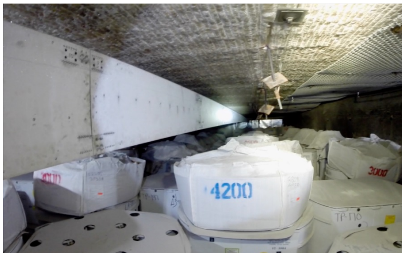
Project Reach's 90-foot boom is positioned over the top of waste containers in Panel 7, Room 7, as a remotely operated video camera collects photographic evidence.
