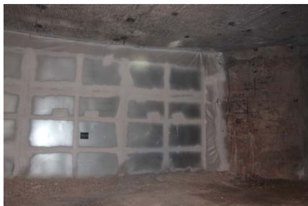
A steel bulkhead seals the entrance to Panel 7, Room 7
