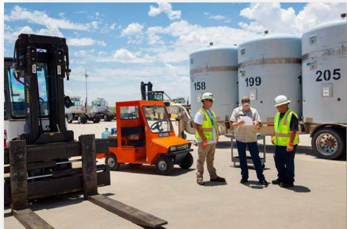
WIPP waste handling personnel review a procedure as part of prestart activities at WIPP.
