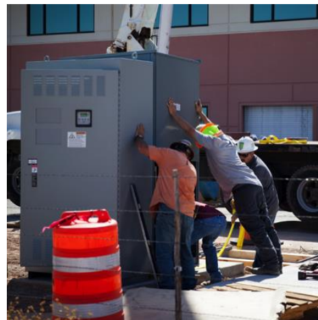
A section of the generator is placed and aligned for installation.
