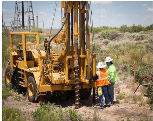
Subcontractors prepare to begin bore hole drilling in support of constructing a new Permanent Ventilation System at WIPP.
