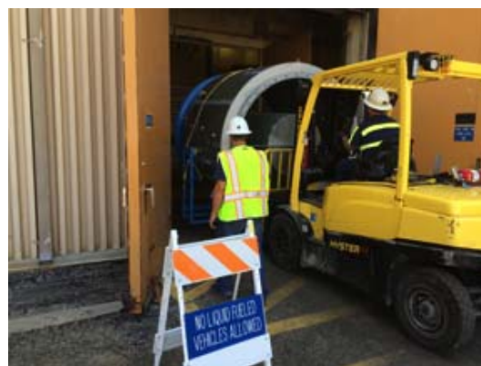
SVS being loaded on the waste hoist.
