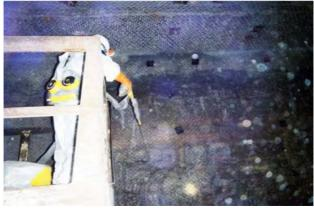
Fig. 1. Underground process for mitigating worker radiological risk using water spray.
