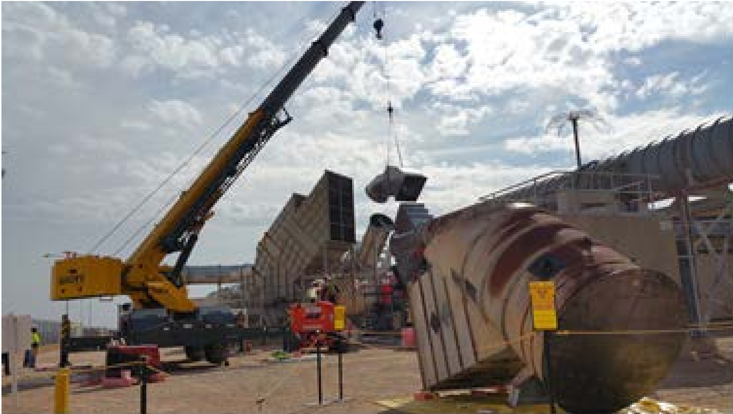
IVS Ductwork Installation Progress
