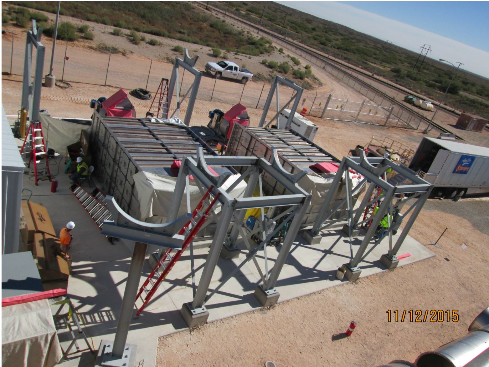
IVS Ductwork Installation Progress
