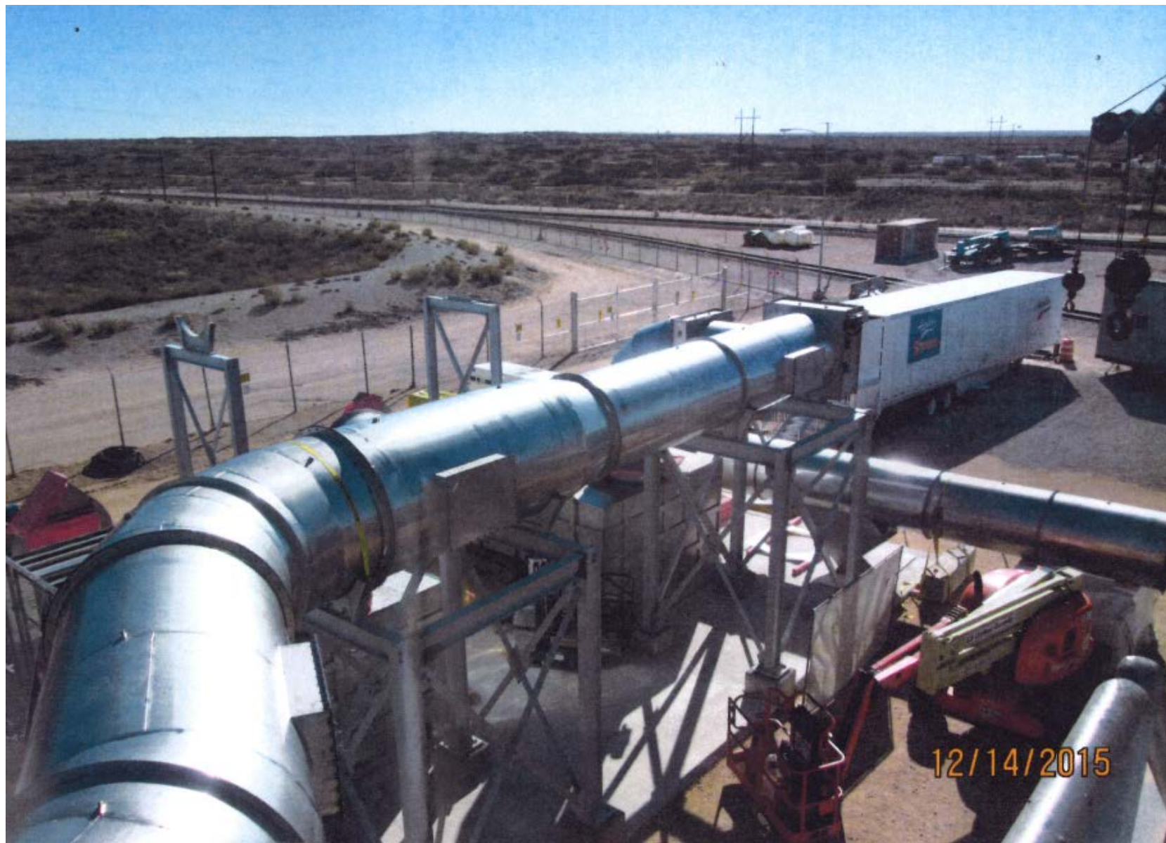
IVS Ductwork Installation Progress
