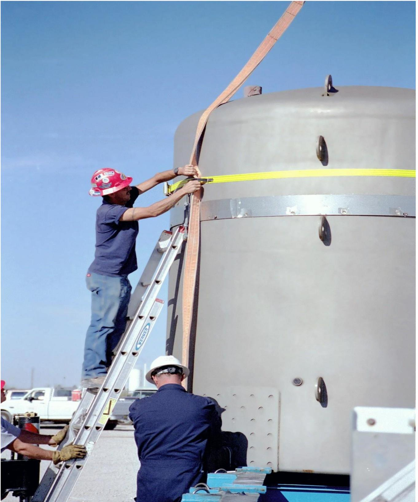
**Figure 2.3-2 –Vertical Lift of a TRUPACT-II Using a Lift Sling Alignment Strap**
