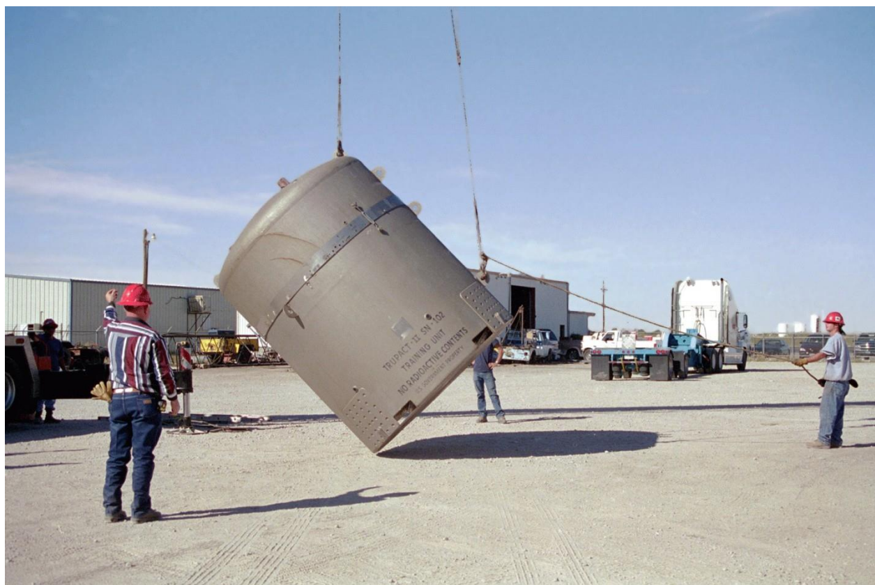
Figure 2.3-15 – TRUPACT-II Package Rotation Using Weld-On Lugs
