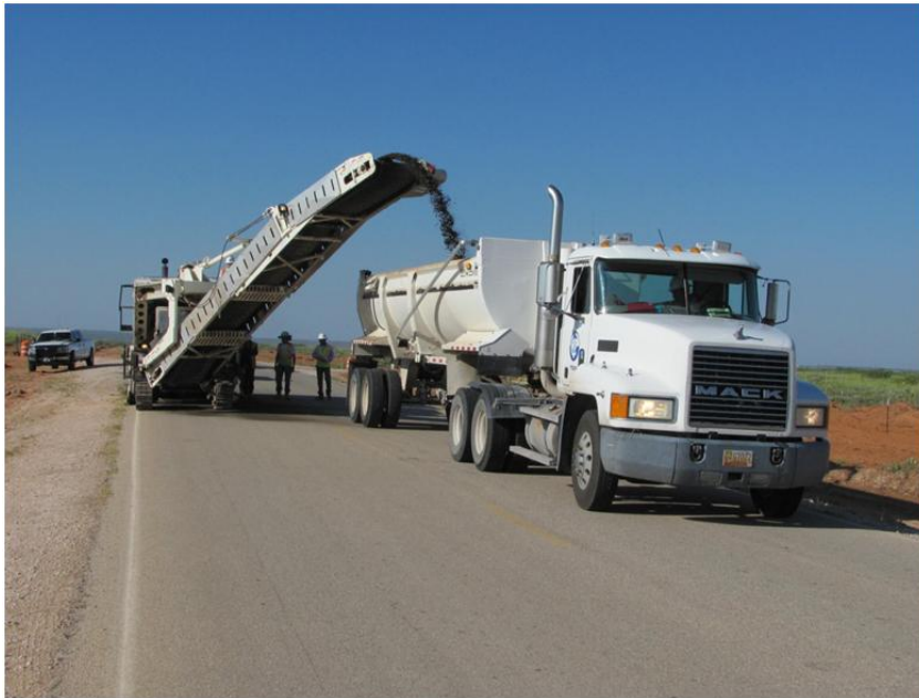
Existing asphalt is milled for recycle and reuse in South Access Road Reconstruction
