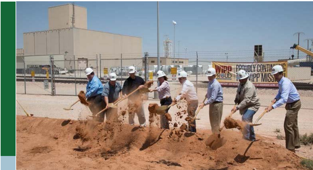
Safety Significant Ventilation System ground breaking
