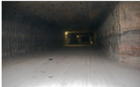
Openings are mined 2,150 feet underground in the ancient salt formation.
