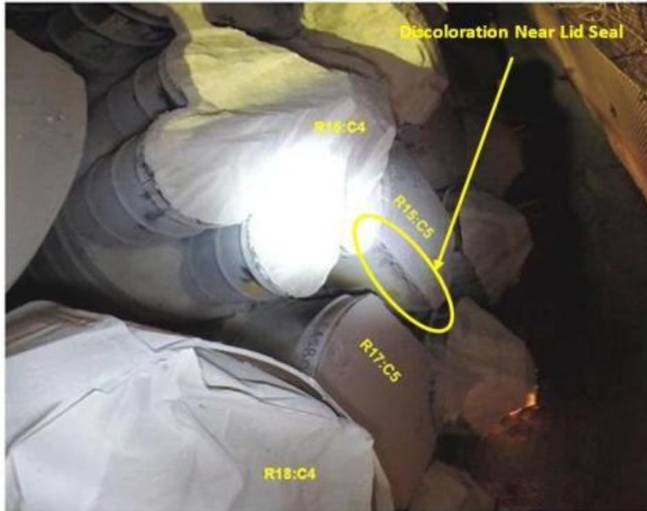
Figure 6-35: Discoloration of SWB at R15:C5
