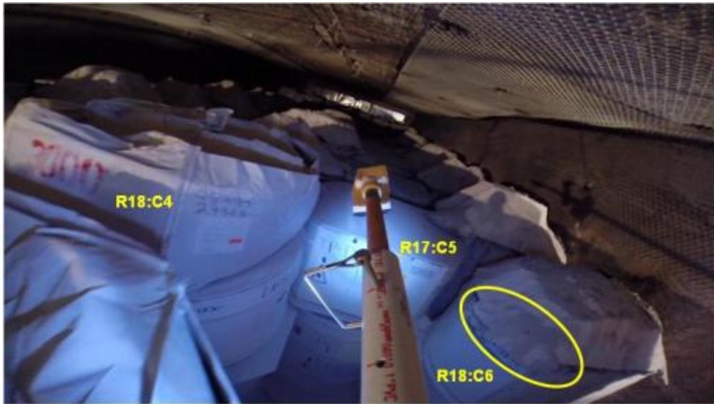
Figure 6-15: Cantilevered Bridge at R18:C6
