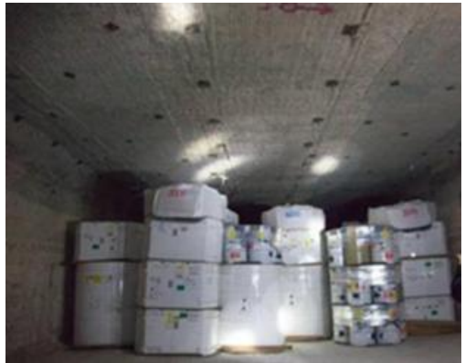
Figure 2-5: Panel 7 Room 7 Waste Face
